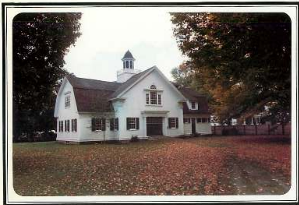
FRONT VIEW OF CARRIAGE HOUSE
